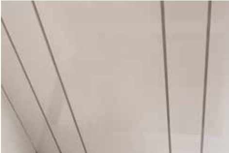
Plain ceiling (no lighting)
